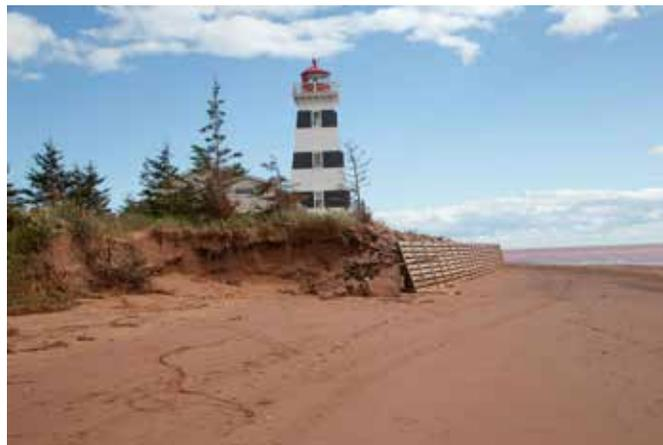
Figure 33. End-scouring on Langley Sea Wall at West Point (D. Jardine, 2019)
