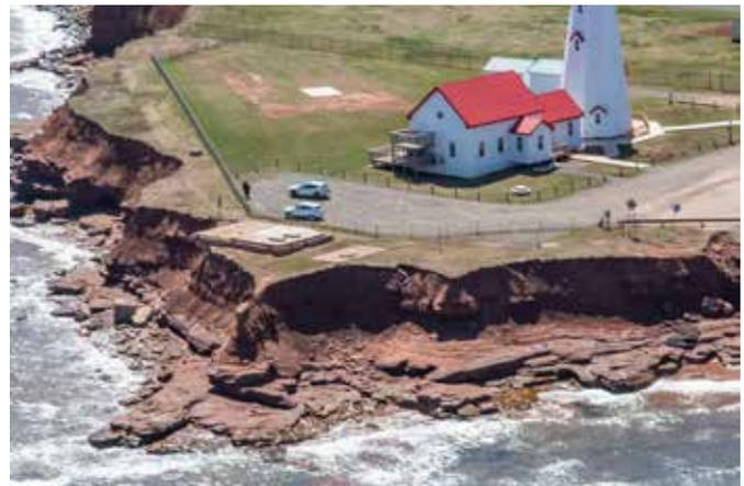
Figure 28. Coastal erosion at East Point where an old foundation is located at the top of the cliff (H. Parnham, 2023)
