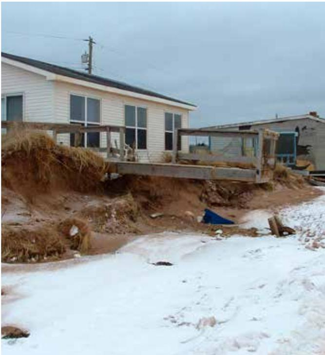
Figure 73. Waterfront cottages damaged in a severe storm event. Maximeville, Egmont Bay PE (D. Jardine, 2006)
