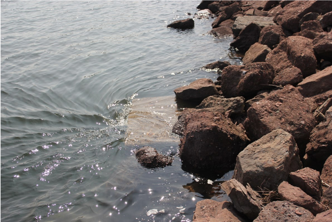
Figure 2. A submerged outlet of Charlottetown’s stormwater system during high tides.
